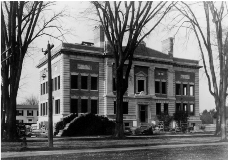
Final construction phase for the Tuck School, May 1904. Courtesy Dartmouth College Library.
