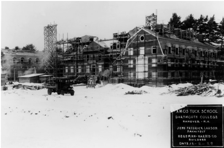
A new Tuck School under construction, December 1929. Courtesy Dartmouth College Library.
