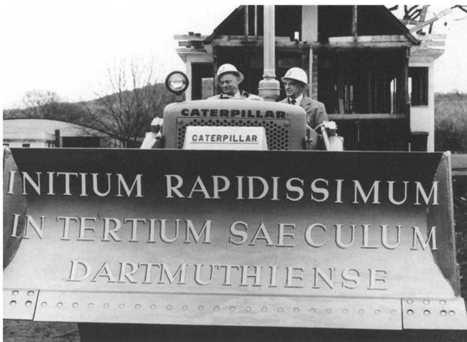
J.S.D. and Mr. Hopkins aboard a bulldozer at ground-clearing for the Hopkins Center, October 24, 1958.
